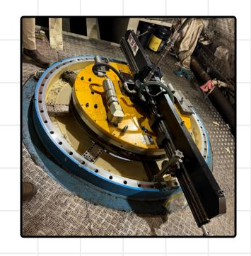
Our team of seasoned professionals is highly trained to perform HOT TAPS (from 1/2" up to 12"), ensuring safe and efficient execution. We use carefully designed, well-maintained equipment to minimize any risk of failure.
